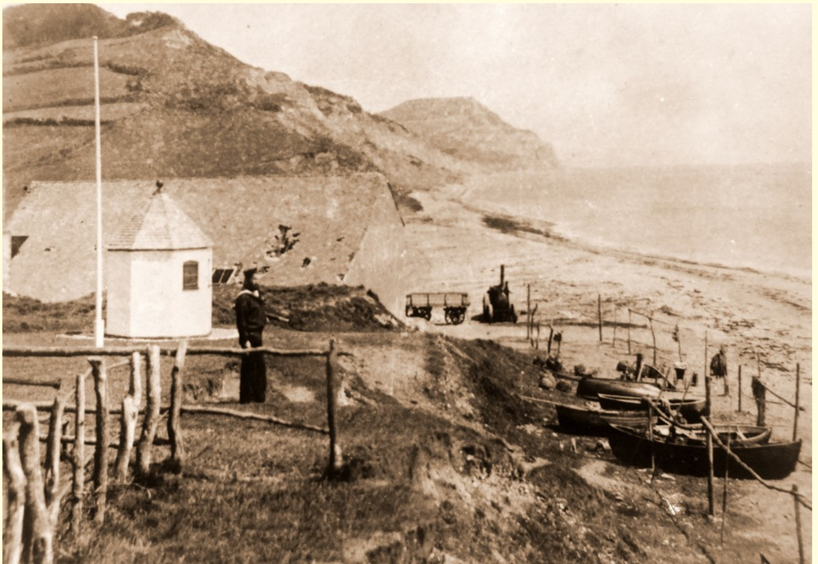
The Cement Factory was built in 1854 for George Morcombe for grinding the lime stones found on the beach for the manufacture of cement. It consisted of a large room facing east with double doors and a small office just inside on the left. Opposite the entrance was a doorway leading into the engine room and to the "boiler room". The engine was a small beam engine with a large fly wheel. This photo was taken by Samuel Hanford who organised the dismantling of the machinery when it was no longer in use for Douglas Pass, the owner.
